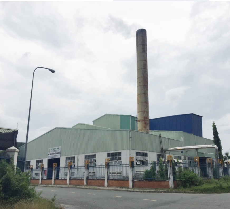
TTG's industrial steam supply factory for Saigon-Cu Chi Brewery in Northwest Cu Chi Industrial Park
